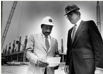
Herman J. Russell consults with Bob Holder in 1983 on construction of Delta Air Lines building in College Park.
